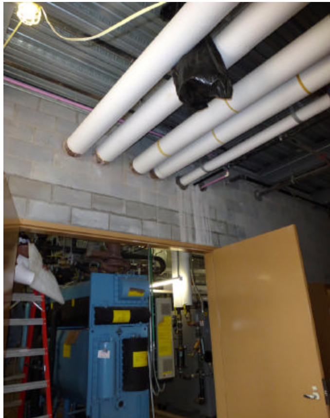
The vapour absorptive machine from China, now dwarfed by the pipes and plumbing that has been installed in the room. It is so crowded in that room, one of the contractors said they had to start assembling from the top of the room and work downwards.
