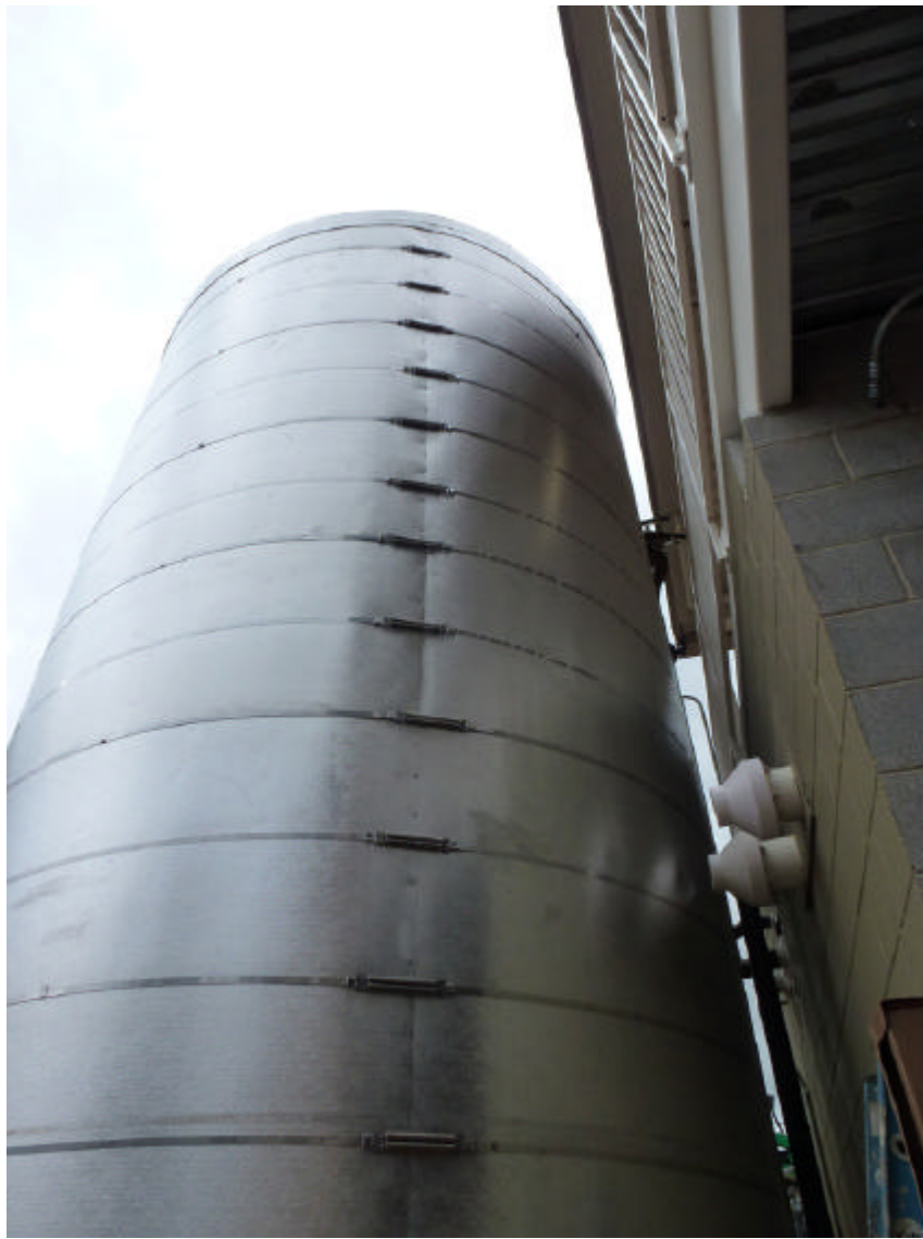
The outside coolant tank looks like it has insulation now.
