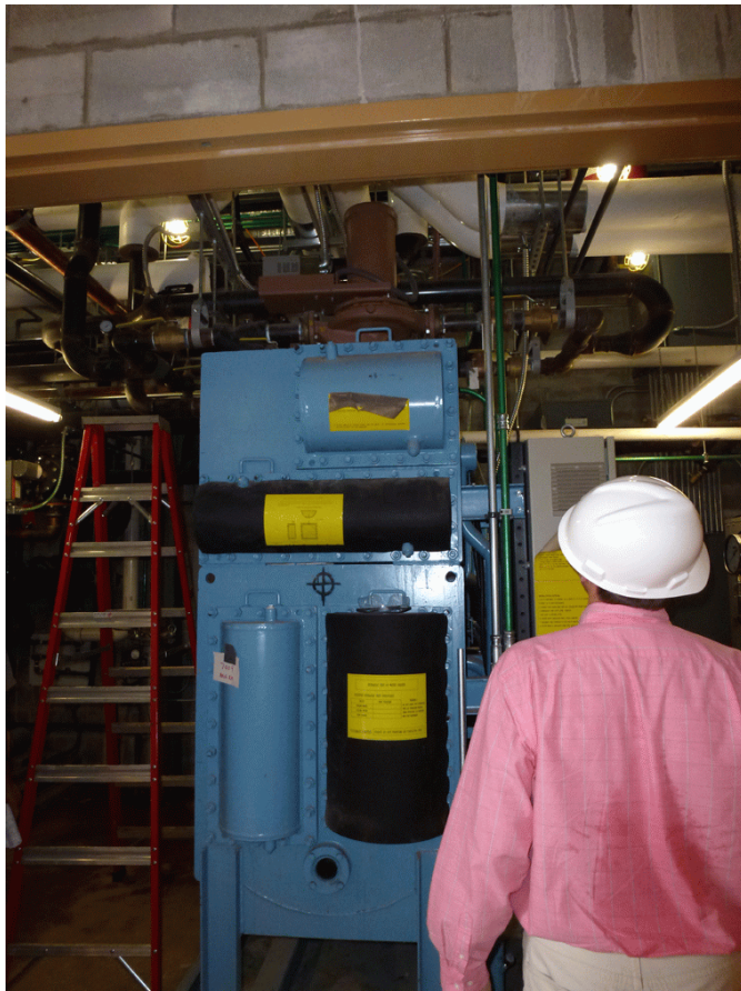
The vapour absorptive machine from China, now dwarfed by the pipes and plumbing that has been installed in the room. It is so crowded in that room, one of the contractors said they had to start assembling from the top of the room and work downwards.
