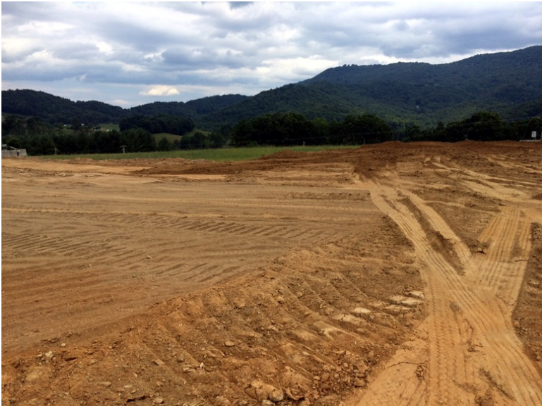
Some of the dome had more dirt to go.
