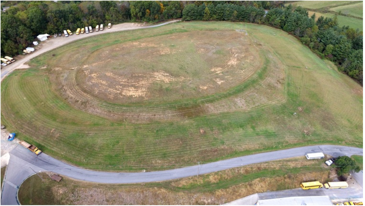
This photo gives the best overall view of the landfill. The methane generator, methane flame burn off device and the leachate pump are located at the upper right of the photograph. Unfortunately, Kris Boyd never mentioned where the EOW markers were in this area of the landfill. Although it looks pretty much to me that everything in this picture is covered by dirt over landfill waste.
