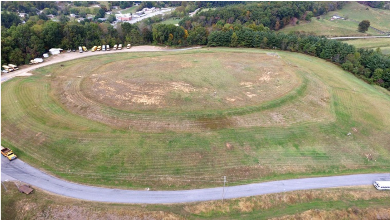
This photo shows the elevations of the mound of dirt on top of the landfill. The paved road passes by the maintenance building and continues around the mound, where some old and surplus vehicles are stored. This is to become the main entrance to the maintenance building. This road continues past the tree line, turns to gravel (which currently the busses cannot negotiate) and is very steep.
