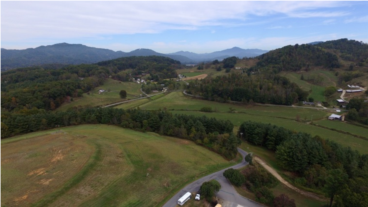
The road leading up to the maintenance building, along with the tree line on the upper side of the road and the drop-off of the mound, are due to be capped, i.e., trees taken down and the road graded and covered with a tarp. This eliminates the main entrance to the maintenance building.
