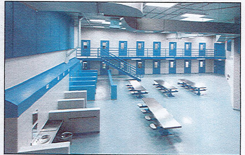
CONTROL ROOM VIEW
