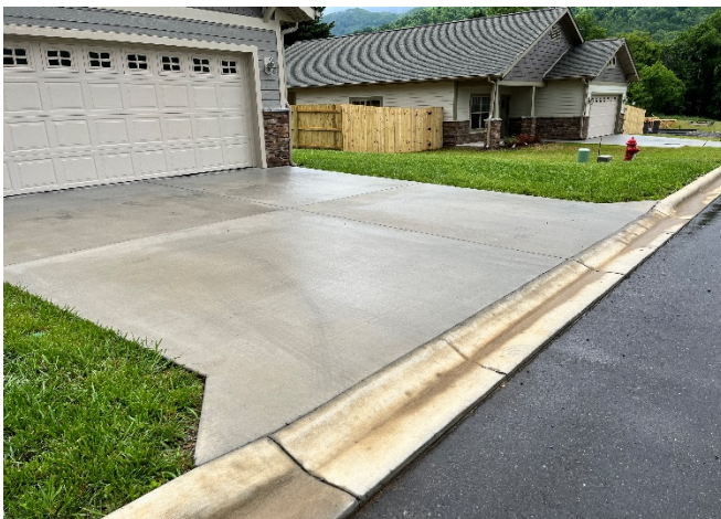
Example of a Good Driveway
