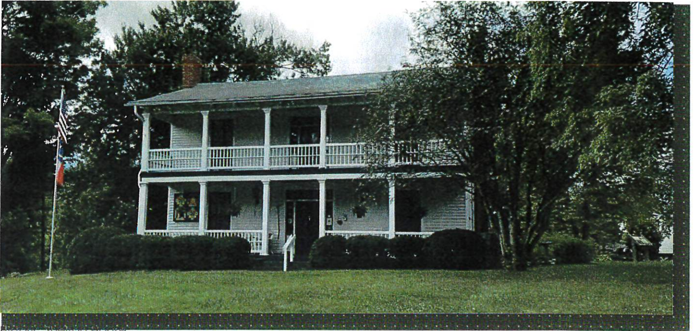
Historic Shelton House
