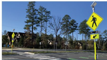
D Dellwood Road Crossing Improvements & Path
