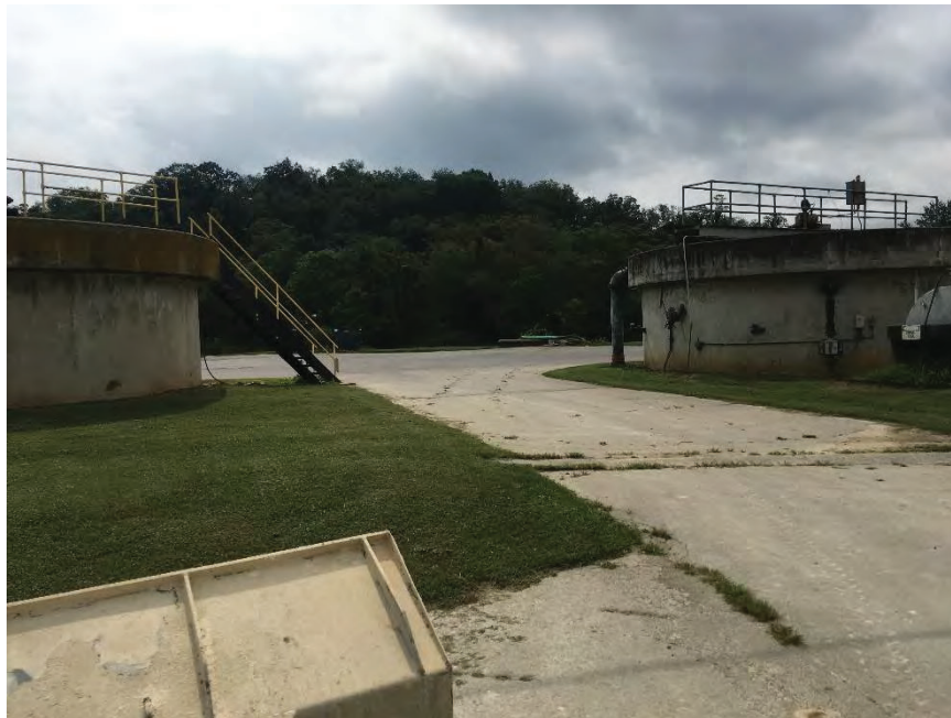
Figure 16. Sludge thickener structures. Concrete is in generally good condition.
